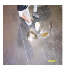
Sprinkle dry sand onto the repair area until the level of sand fills the hole and levels the repair area until level with rest of the floor surface.
