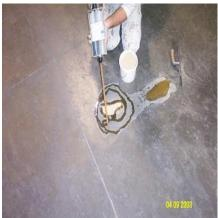
Apply a thin layer of the mixed liquids from the cartridge set onto the concrete. For larger areas, it may be beneficial to use a small brush to spread the liquids to evenly cover the repair area.
