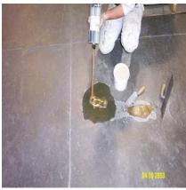
Then saturate the sand with the liquid. Reapply more sand and liquid as needed until the area is built up level to floor.
