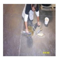
Finally, trowel the floor to smooth out the area and remove any excess material. Allow the material to cure for ten to twenty minutes before foot traffic. Immediately after you are through using the liquids from the tube set, remove the static nozzle and place the end caps back on each tube as this will allow the use of the tubes for later repairs. For heavy equipment such as fork trucks, allow the material to cure for a half hour to an hour before using area that has been patched.
